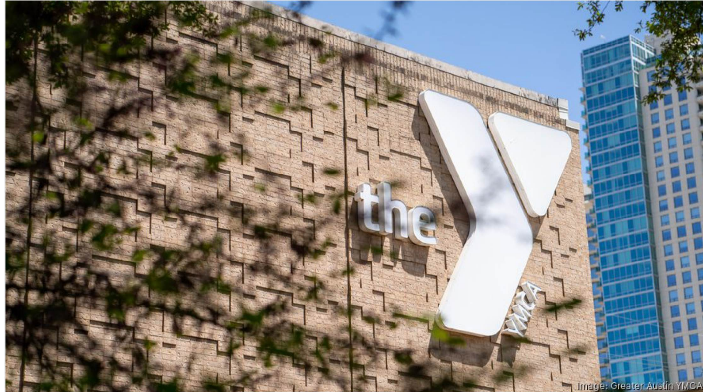
The exterior of the Townlake YMA, which could be redeveloped to add a new facility and housing. GREATER AUSTIN YMCA
